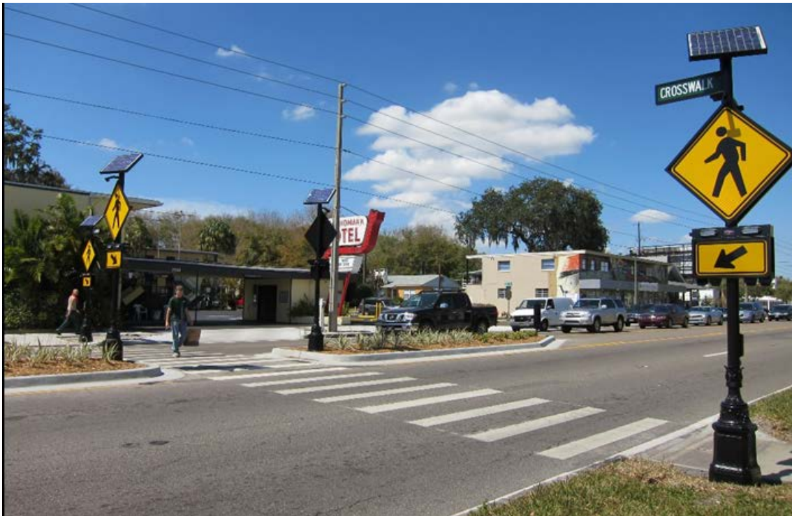
4th Street North, St. Petersburg, Florida
